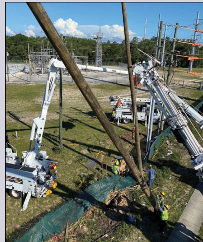
WREC crews at work
