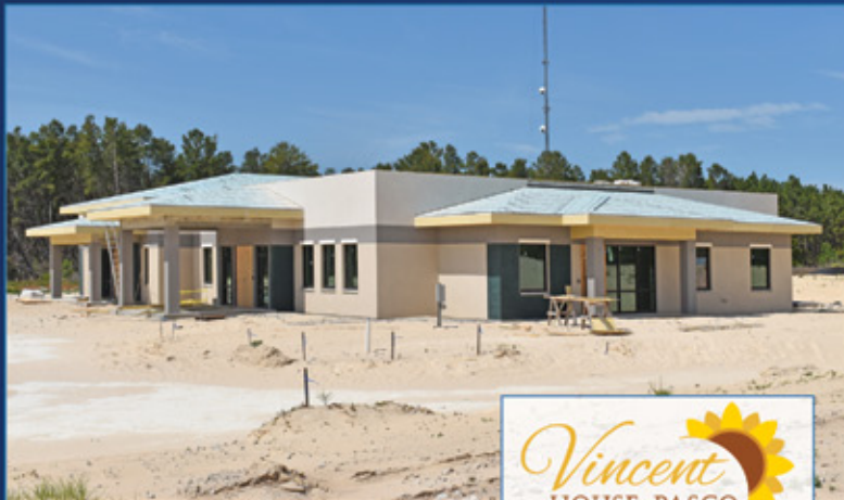
New Vincent House - Pasco under construction
