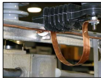
ARRESTOR GROUND DETAIL VIEW
