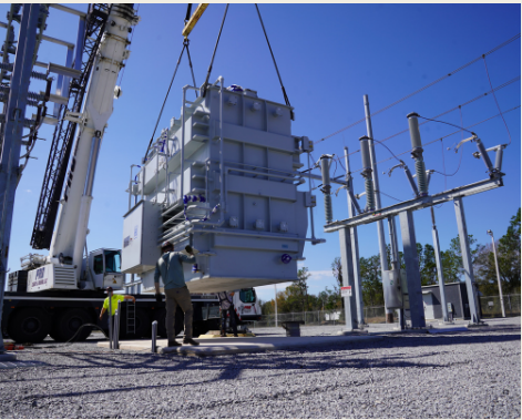
Transformer being delivered to new substation.
